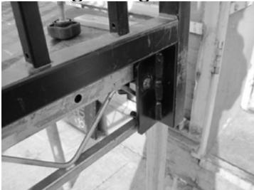
3. Fit the backplate over the pin of the guardrail.
